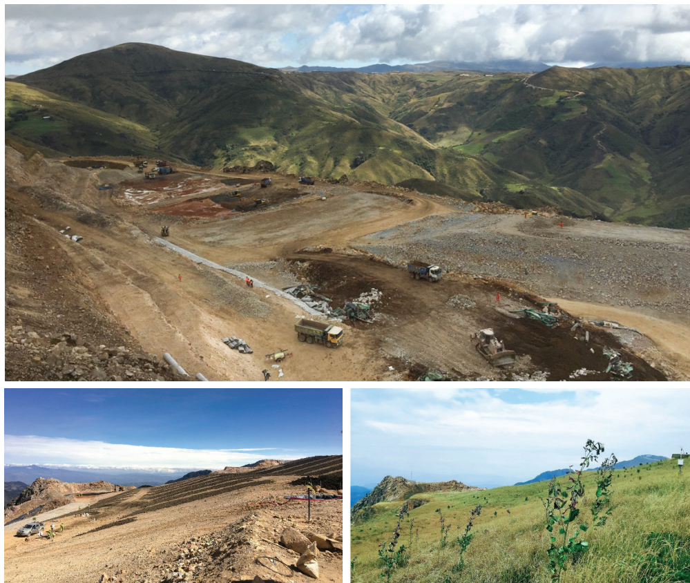
Figure 1 Site view before (above), during (lower left) and after (lower right) cover implementation.
