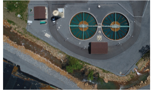
Figure 4 T & T AMD treatment plant (image: Chester Wright, OSR)
