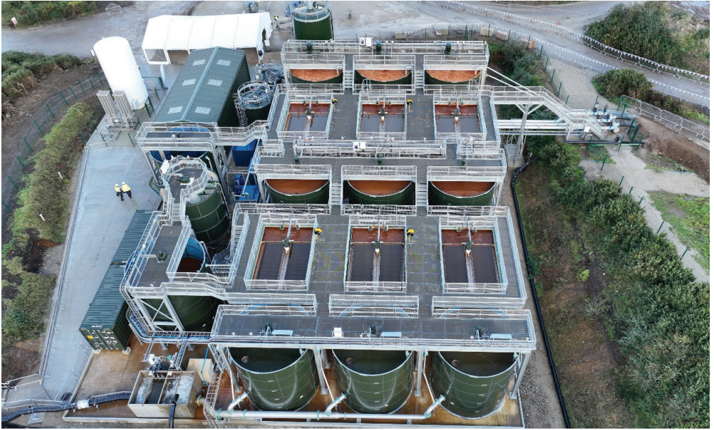
Figure 5 South Crofty MWTP – 26 th October 2023 Stage I in the Background
