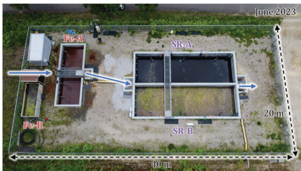
Figure 1 Large-scale multi-step passive treatment test system (image: Yusei Masaki). Fe-A and Fe-B: Fe-oxidizing/removal biochemical reactors A and B; SR-A and SR-B; sulfate-reducing biochemical reactors A and B. Blue arrow indicates the direction of flow
