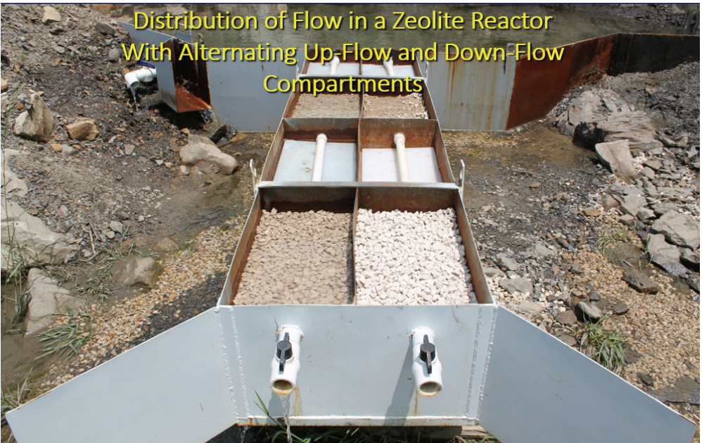
Figure 2 Distribution of flow in a zeolite reactor with alternating upflow and down-flow compartments
