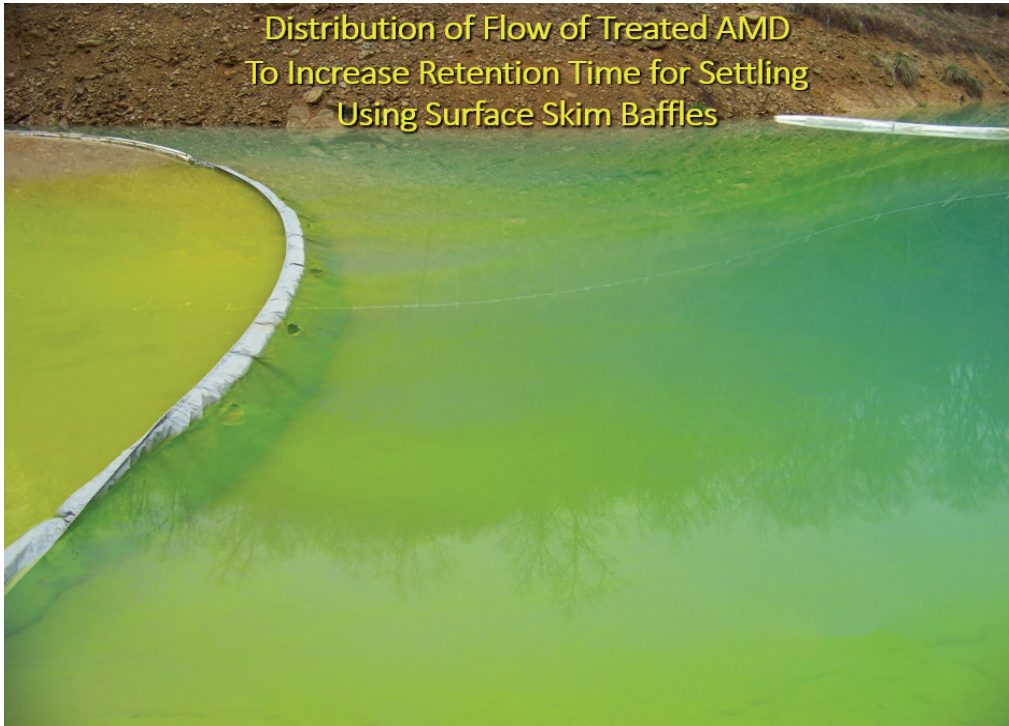
Figure 3 Distribution of flow of treated AMD to increase retention time for settling using surface skim baffles
