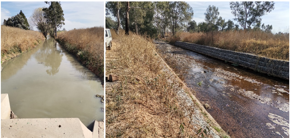
Figure 3 Completed earth canal with a downstream gabion wall
