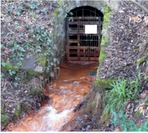
Figure 1 Water-bearing adit in the southern Ruhr area (image: THGA).
