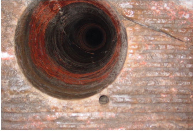
Figure 4 Exploration borehole intersects a fracture exposed in the roof at the sylvinitic mining level, Solikamsk mine #3.2004).
