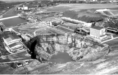
Figure 2 Large collapse structure occurred at Berezniki mine #1 in 2007 after the water influx initiated in 2006. The size of structure achieved 446 to 335 m in 2009. Sinkhole cut the railroad Perm - Berezniki that is seen in the front of sinkhole (Berezniki 2009).
