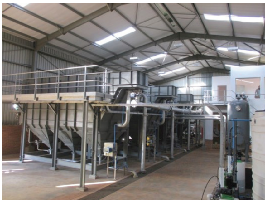
Figure 1 – Dissolved air flotation units inside the WRP
