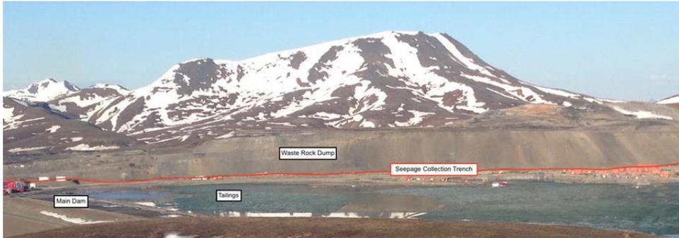
**Figure 9** – Tailings facility and waste rock dump
