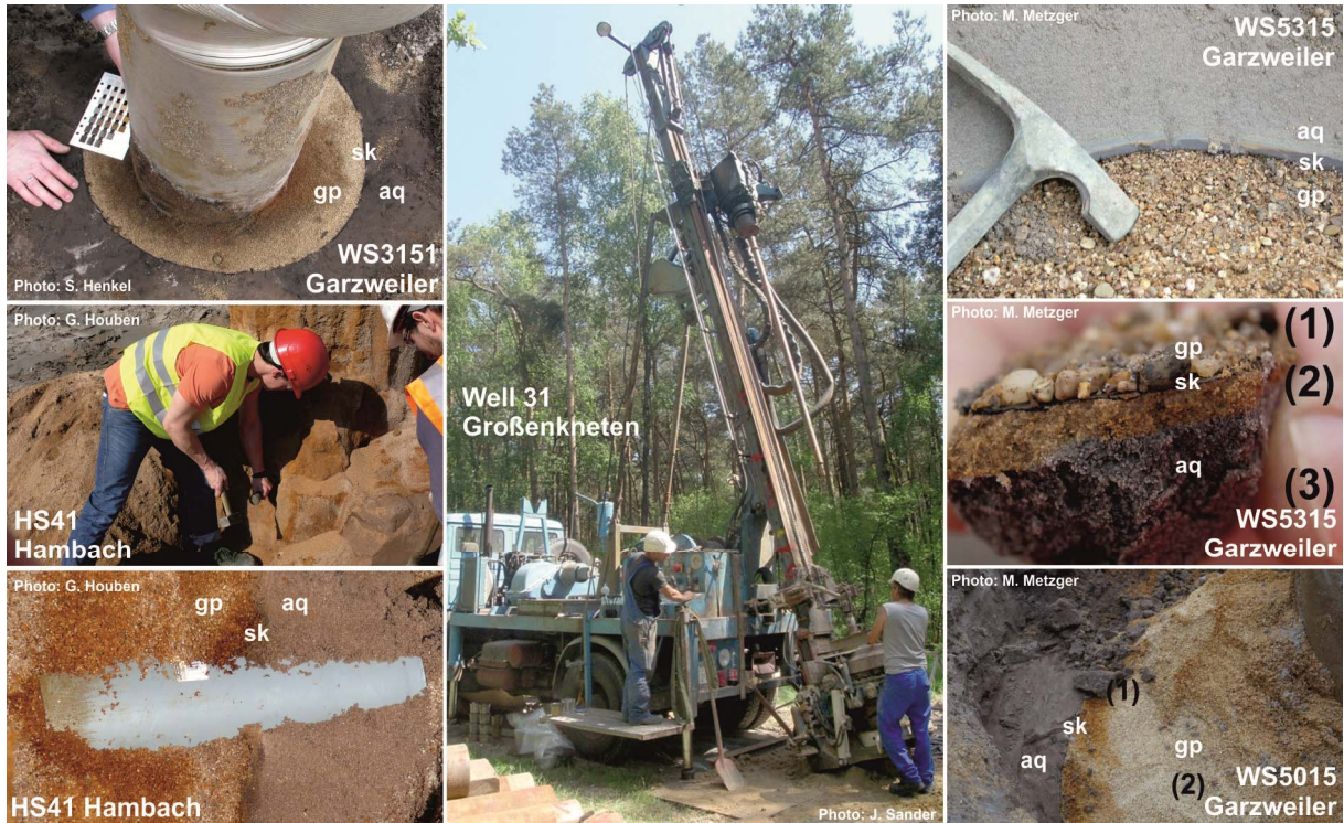
Figure 1 Inclined drilling into the annulus of a decommissioned water supply well in Großenkneten (centre) and undisturbed sampling at excavated open-pit dewatering wells in the lignite open-pits Garzweiler and Hambach (left and right).
