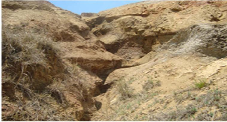
***Fig. 4*** Devastating effects of erosion in the tailings dump
