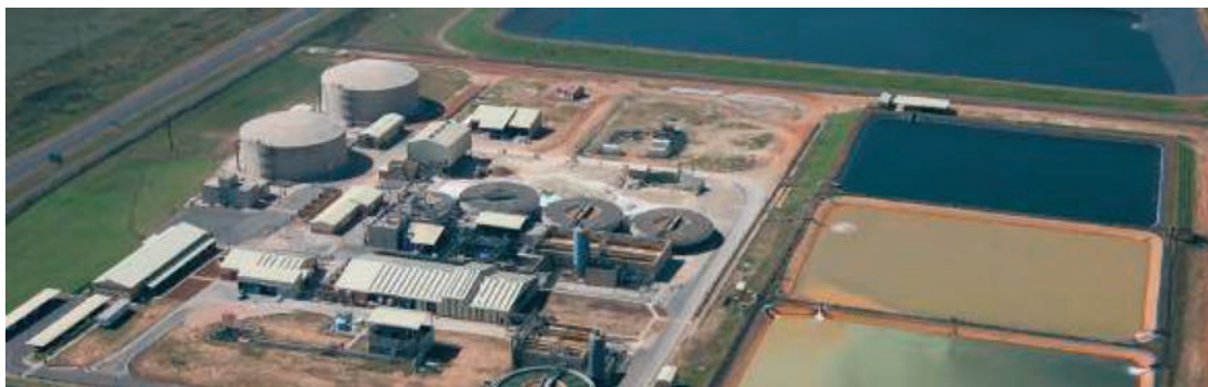
Fig. 1 eMalahleni Water Reclamation Plant, South Africa
