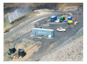
Fig. 5 Pit dewatering site installation
