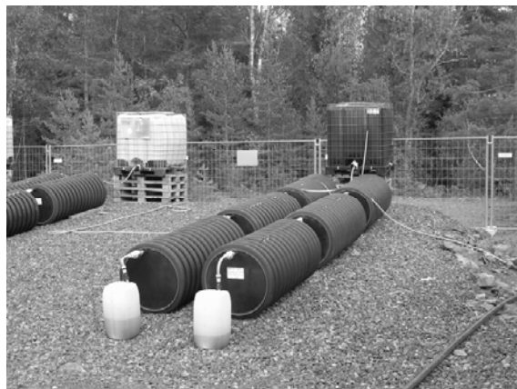
Figure 1 View of two of the filters and the ARD reactors. Each filter consists of three coupled plastic barrels (each 0.5 m 3 )
