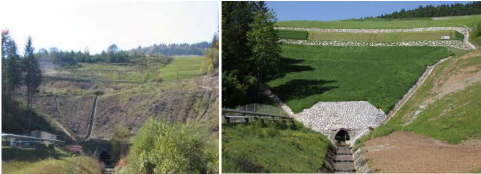
Figure 1 Eastern slope of the mine waste rock dump Jazbec prior to (2005) and during remediation (2008).
