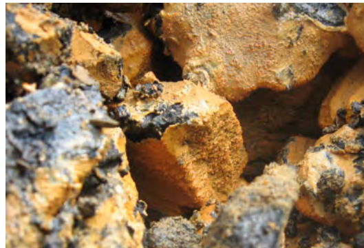
Solids form scale on limestone
