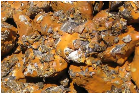
Scale flakes off revealing clean LS surface
