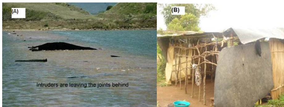
Photograph 3. Vandalised contact water storage facility with liner stolen (A); Liner pieces are used as local building material (B).
