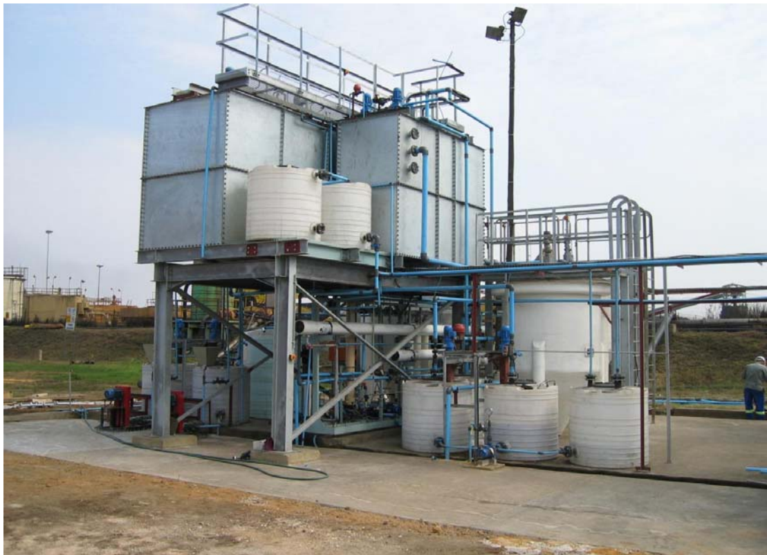
Figure 2. 4.5 m 3 /hr Demonstration Plant
