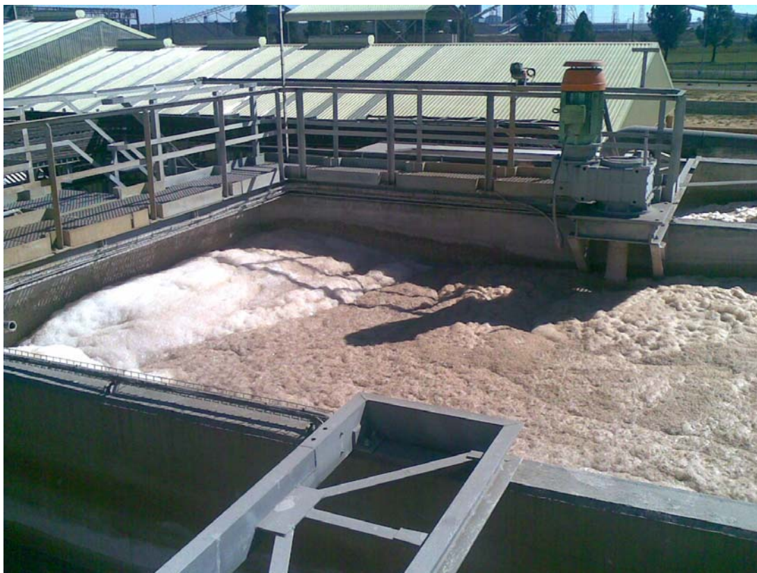
Figure 13. Foam in the Precipitation Reactor
