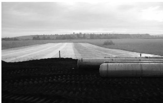
**Figure 9 Laying of sealing material with tracked vehicles**
