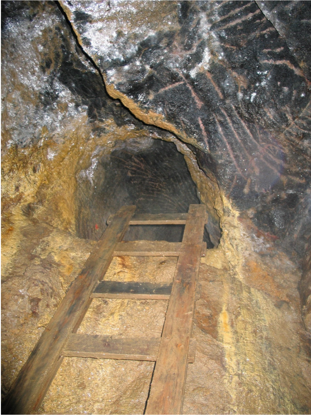
Supplement 7 An example of manually stoped-out adit from the 16-17 th centuries
