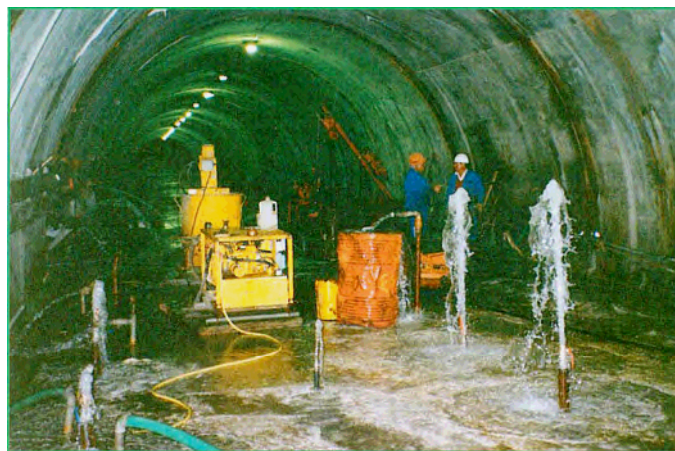
Picture 1 Injection process at the inspection gallery
