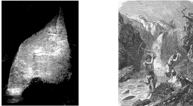
**Fig 2.** Exploitation by the “*ruina montium*” method in Las Medulas and works for disintegration of auriferous alluvium.
