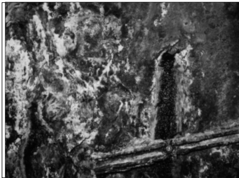
Figure 5. Efflorescent mineral buildup along fracture plane intersection with tunnel wall
