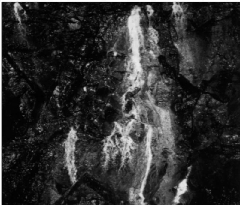
Figure 6. Sulphur oxidizing bacterial slime at groundwater inflow points
