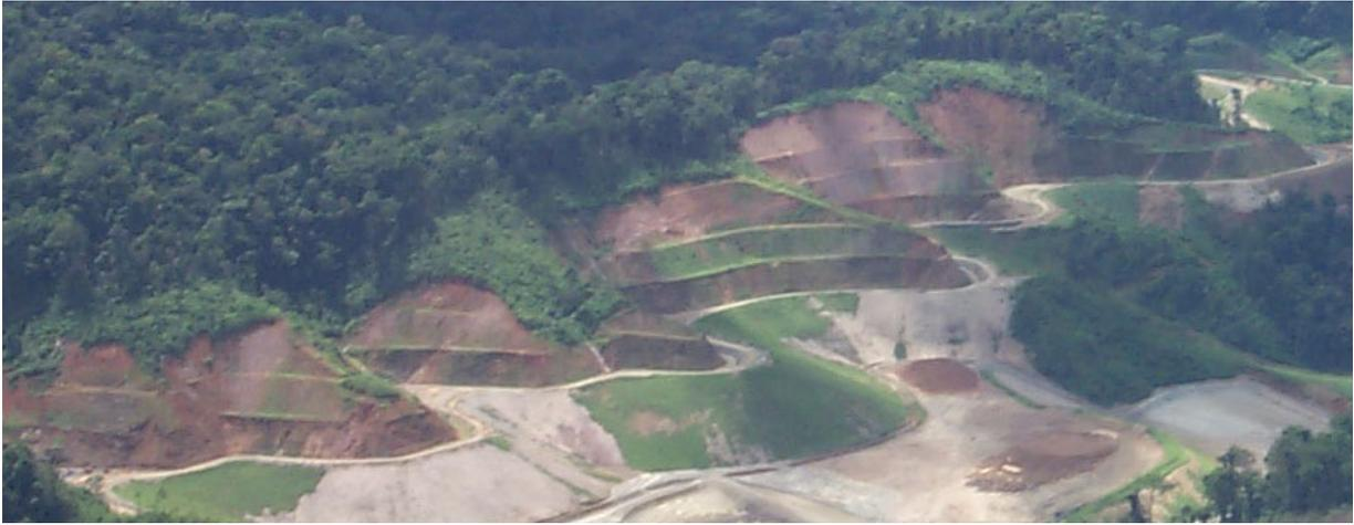
Photo 2: Channel with moderate slopes and side cast material.
