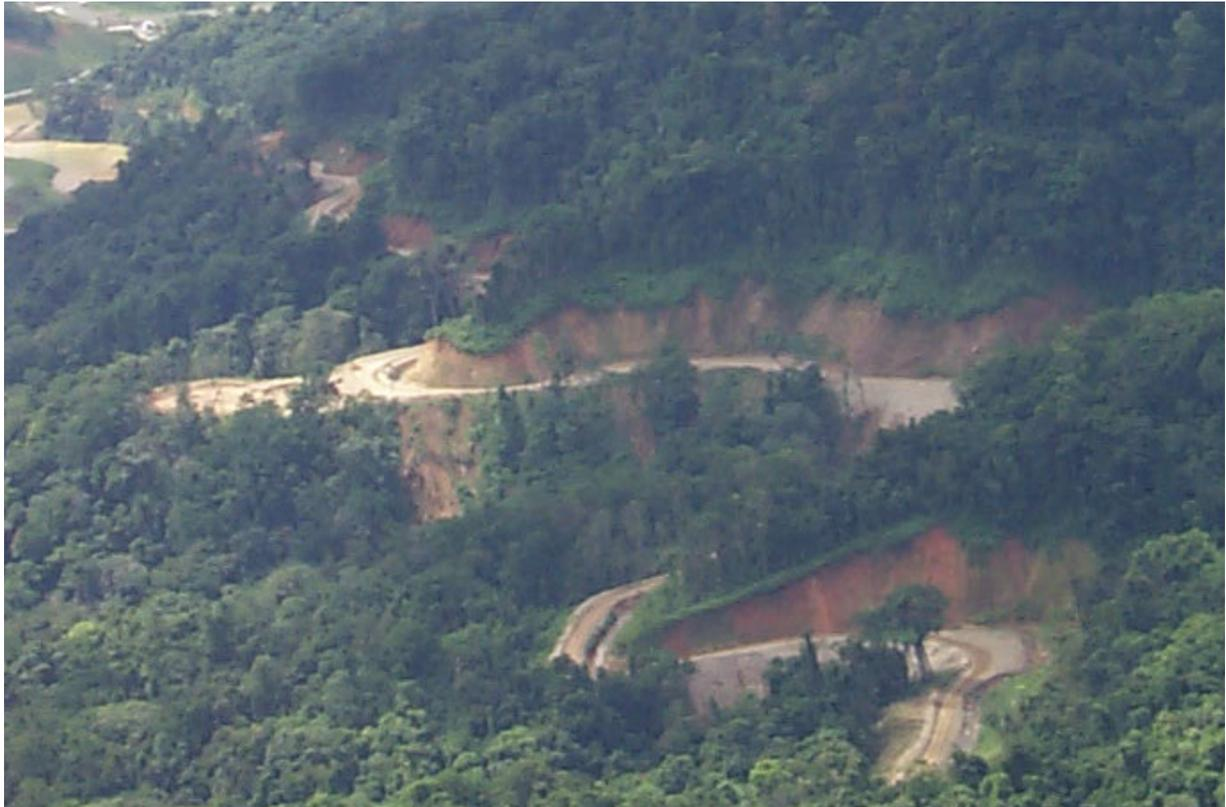
Photo 1: Channel with steep slopes and side cast material.
