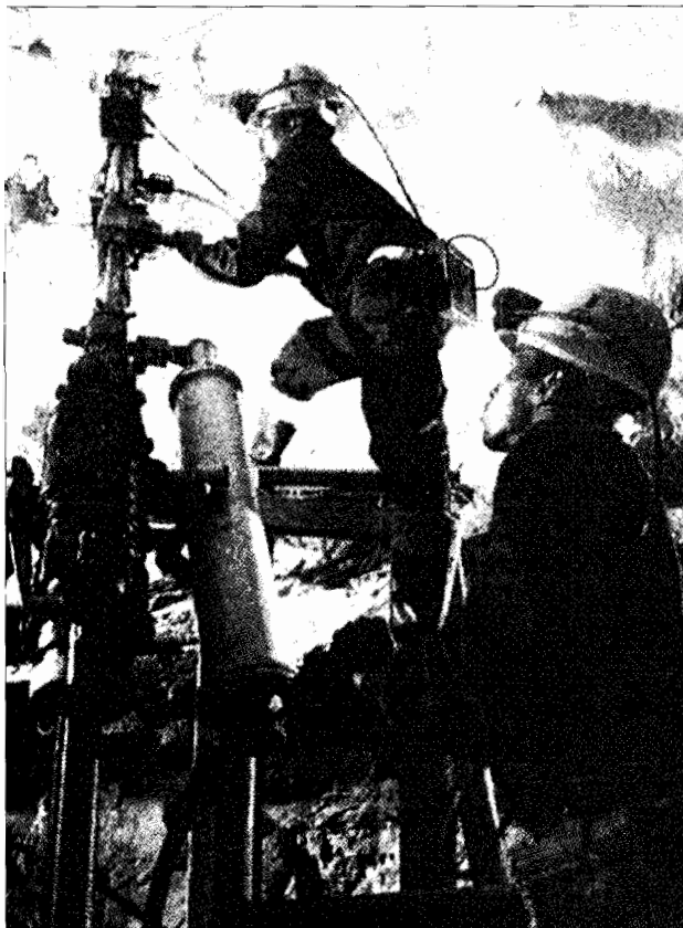
Figure 3. Drilling underground with a Kempe U39 machine.
