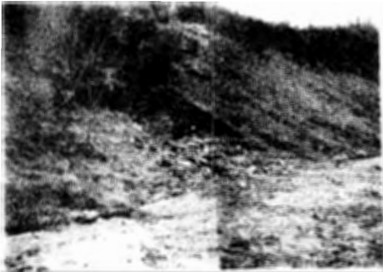
Figure 4: Boccheggiano Mine, Central Italy. Cavity inside the dam of the tailings pond that is appeared in consequence of the breakdown of its roof during the 1998 earthquake, above, and that has been on purpose filled, after its widening for overtopping, below.
