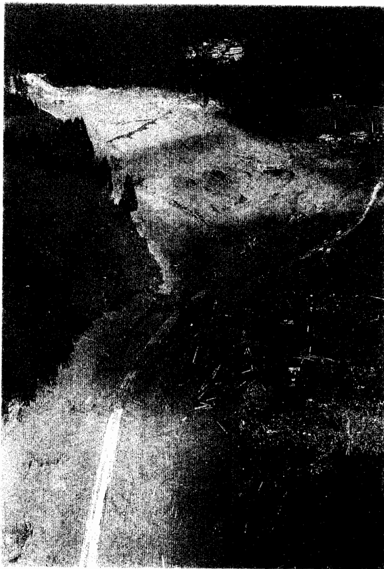
Figure 7: Prestavel Mine, North-Eastern Italy. The mud, that came auto from the tailings ponds, poured into the Fiemme Valley, crossed the Stava Torrent, on the left, and destroyed and buried the village of Stava which had been built in the lower on the right area of the figure.
