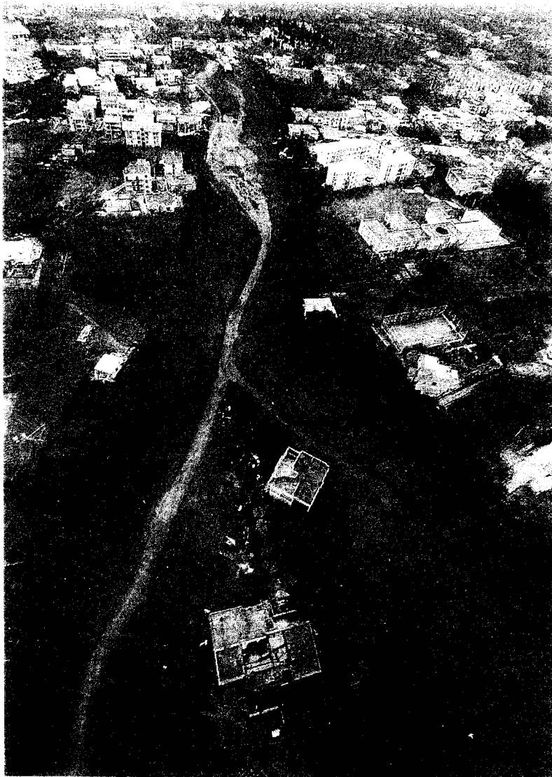
Figure 9: Flow slide of Sarno, Southern Italy. Mud flows which have destroyed and buried a quarter (Anon, 1998).
