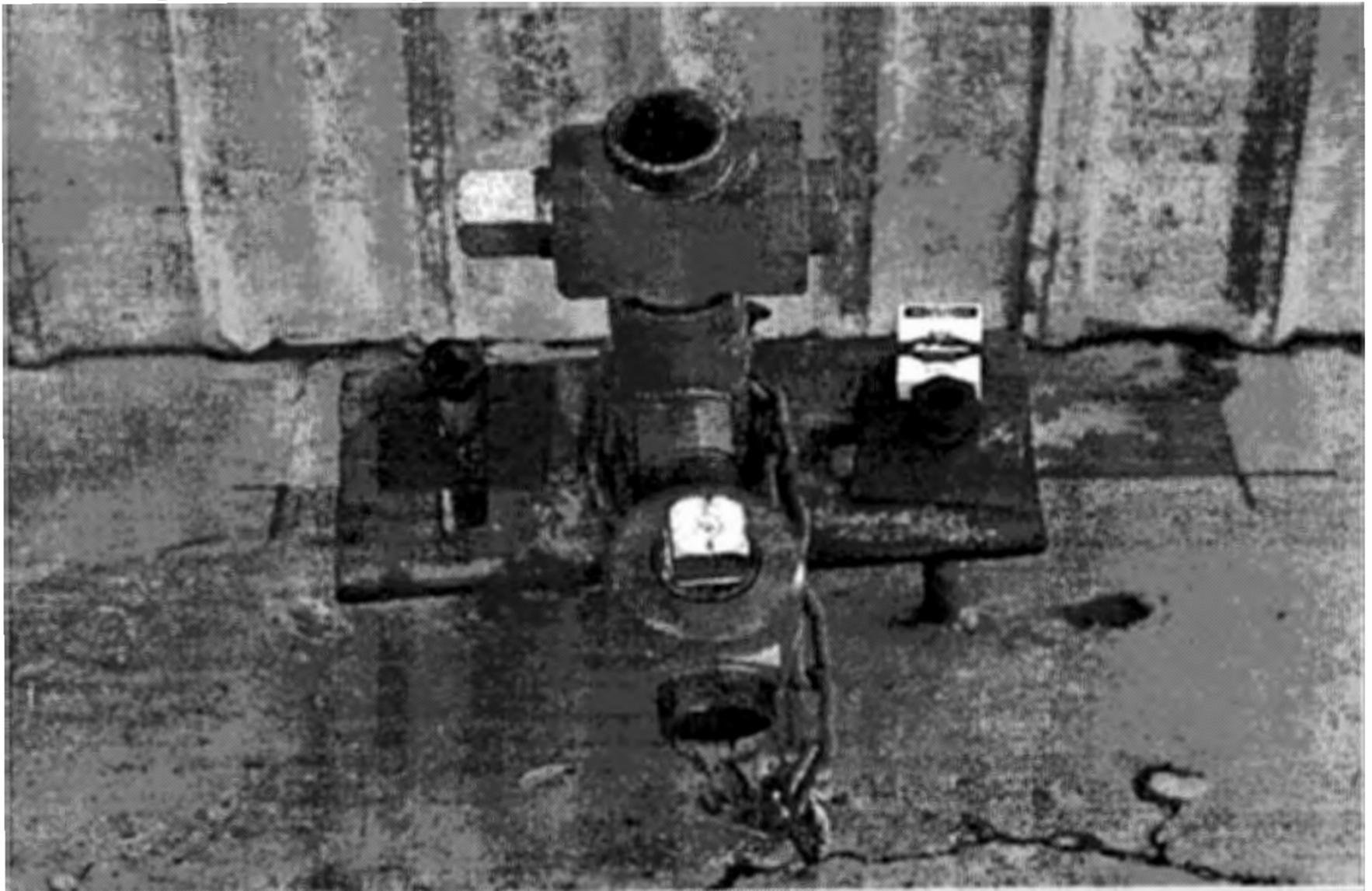
**Photo 3: High Pressure Safety Valves. Front view.**
