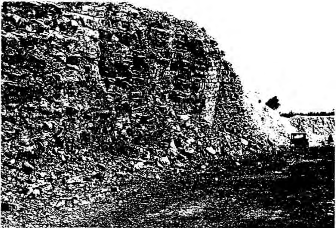
Photograph No 8 Bench B, N zone/W wall. Toppling failure
