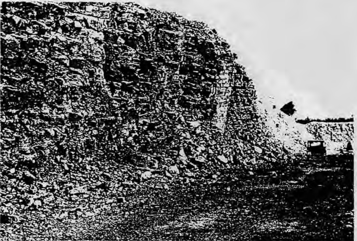
Photograph No 8 Bench B, N zone AM wall, Toppling failure reproduced from best available copy
