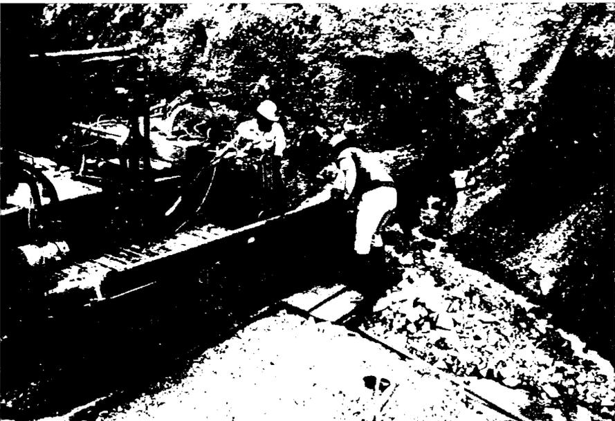
Figure 8. Aardvark Drilling Drainage Hole.
