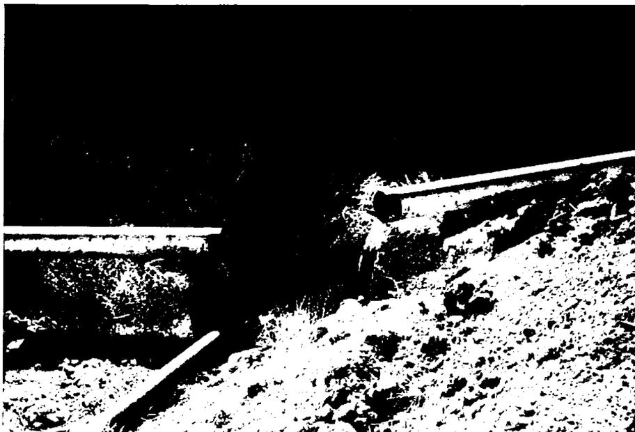
Figure 12. Water Collection System Discharging to Pump Sump Intake.
