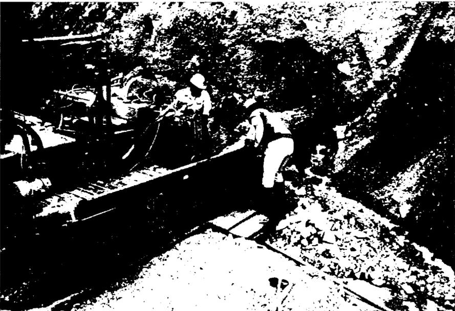
Figure 8. Aardvark Drilling Drainage Hole.
